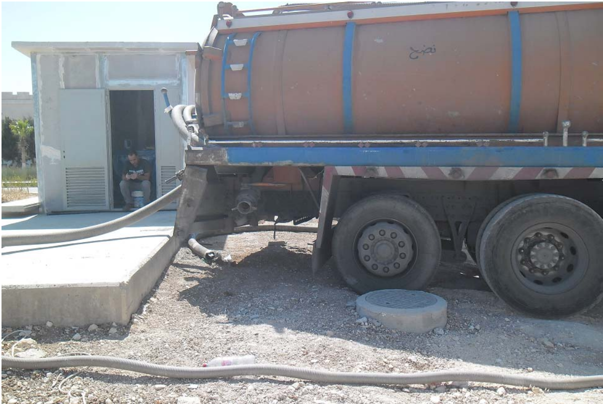
Evacuating & Cleaning of underground tanks at the Inlet Structure
