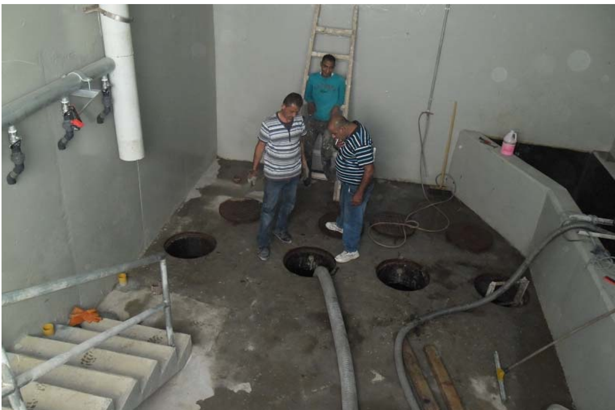
Evacuating & Cleaning of underground tanks at the Inlet Structure
