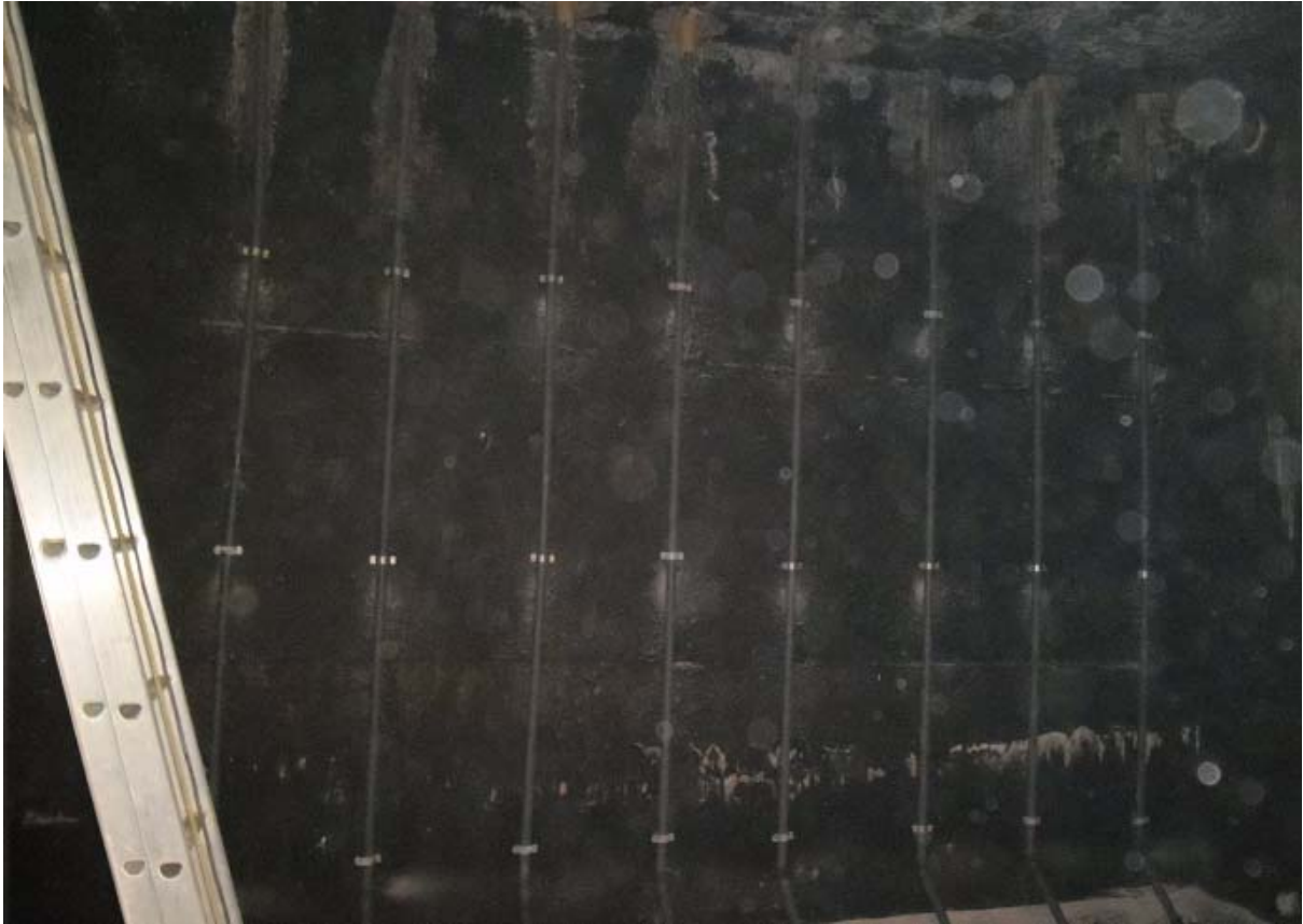
Air Diffuser lines inside the Balancing Tank
