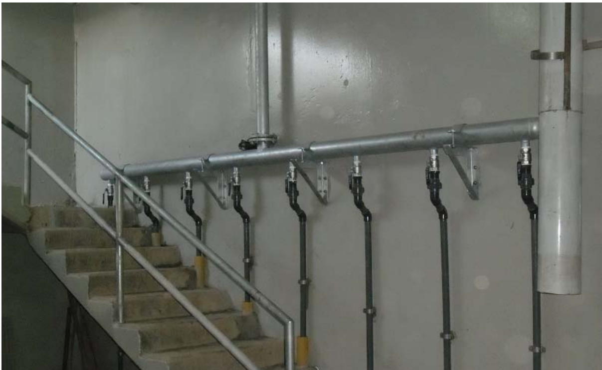
Aeration System at the Balancing Tank
