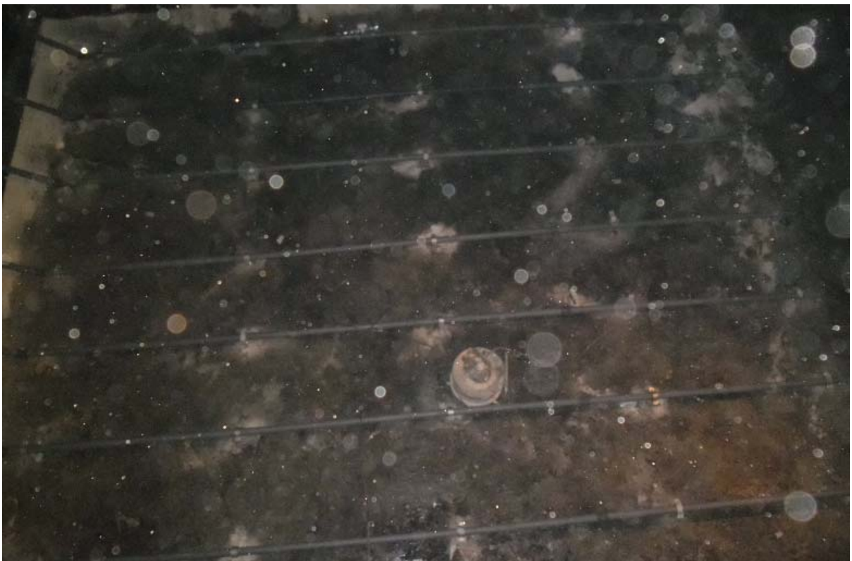
Air Diffuser lines inside the Balancing Tank
